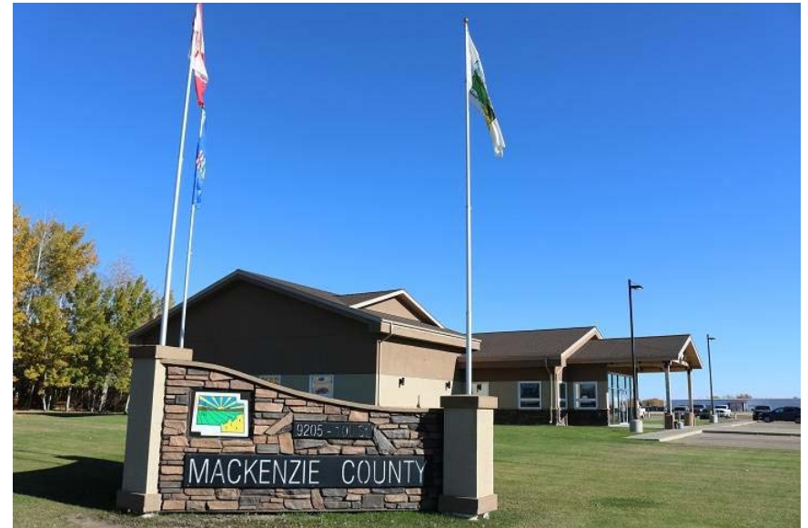
La Crete County office
